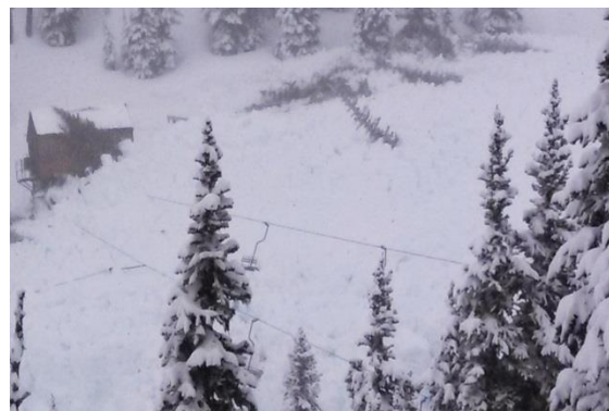
Figure 5: The two-story bottom terminal of the lift hit by the avalanche from The Throne on March 10 th . The avalanche came from the right.
